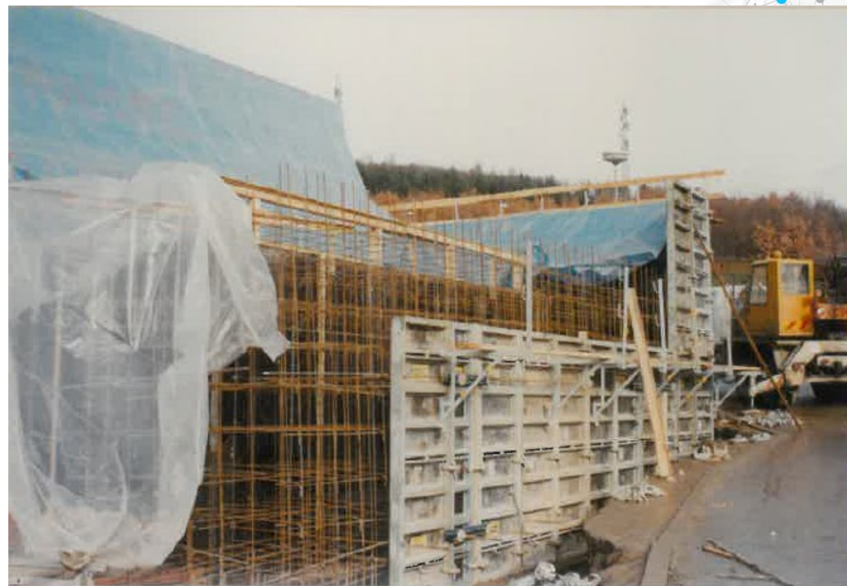
30.1.1999 – reinforcing the walls
