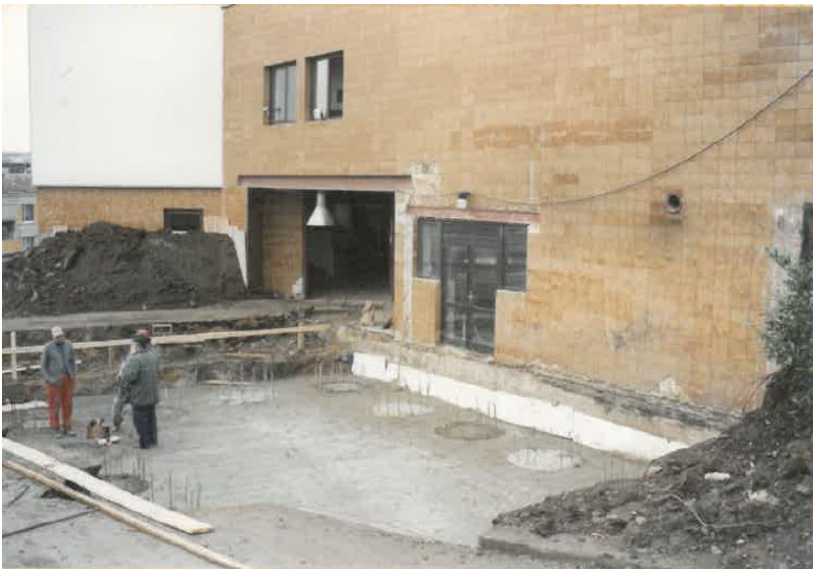
17.12.1998 Future vault The bearing piles are 14-16 meters deep
